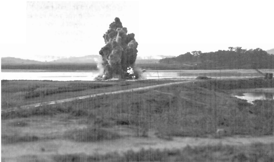
KUM RIVER BRIDGE EXPLOSION
